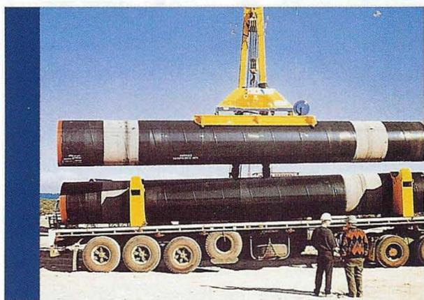
**A 9.6 tonne pipe being unloaded by a Vacuum Lift unit attached to a mobile crane.**
