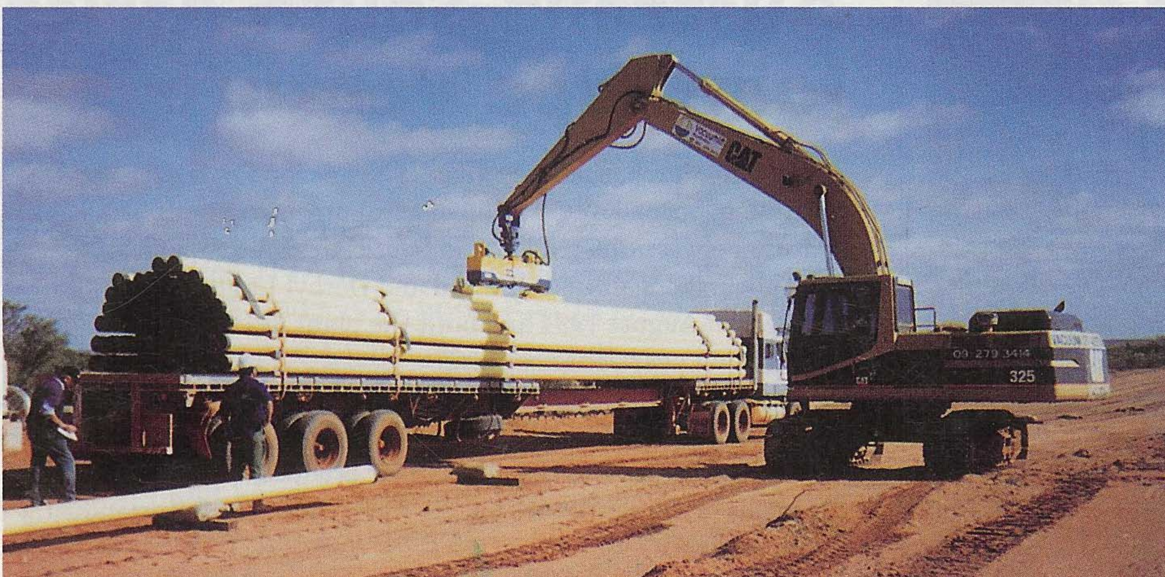
Vacuumlift Australia's excavator / pipehandler unloading pipes on the Moomba - Sydney pipeline.
