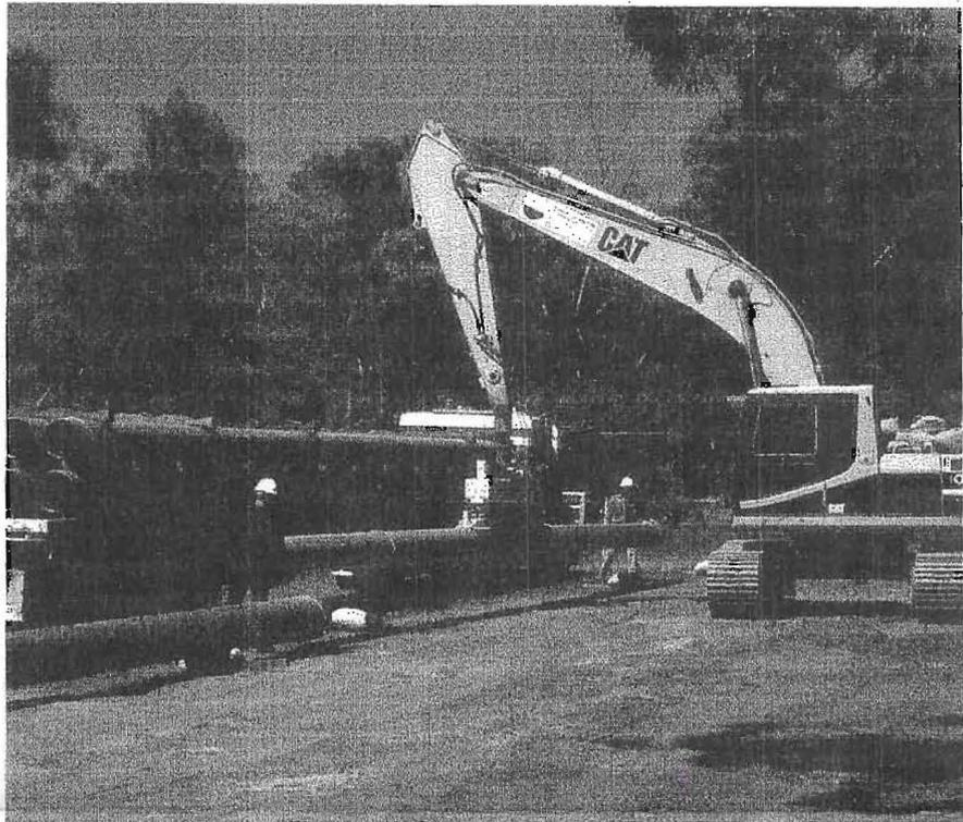
A vacuum lift is used to lower pipe to the ground to avoid damage to
